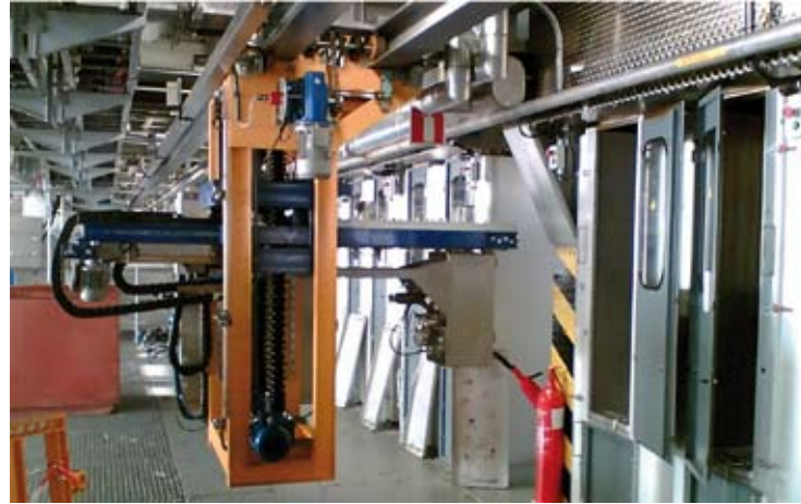
Robotised system of exchanging heads in stoves.
