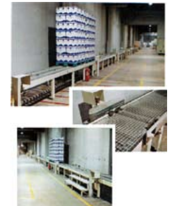
Roller conveyor belt.
