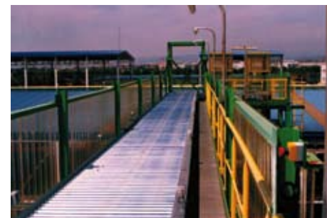
Roller conveyor belt.
